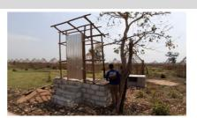
The toilette: there is a WC unit every two shelters. The basement is made by CHB. the structure by wood and the roof by corrugated iron sheet.
